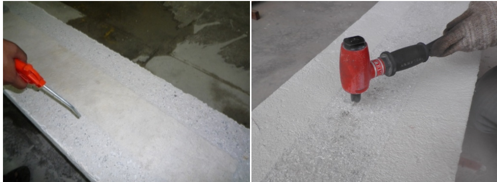
Fig. 1. Preparation of surface
