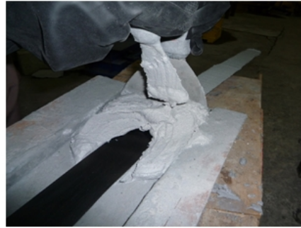
(b) Placing of adhesive on CFRP laminate
