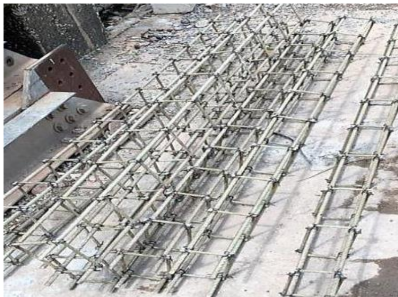
(c) Fabricated GFRP cages
